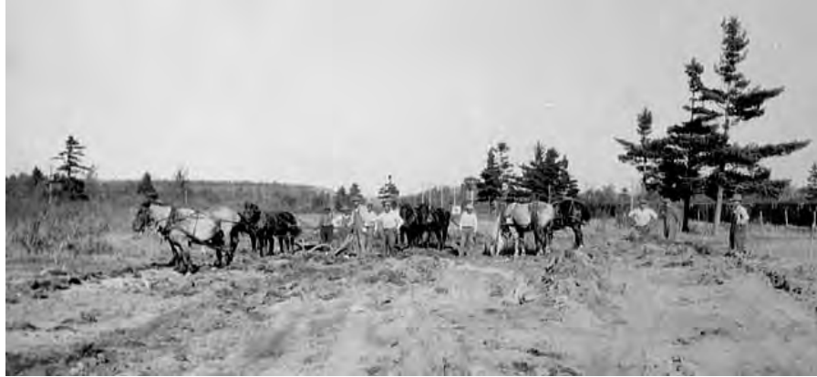
Figure 36. Highway 35 construction in 1933 near Aurora.
