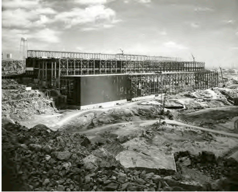
Figure 45. Erie Mining Company Concentrator Building Construction, ca. 1954.
