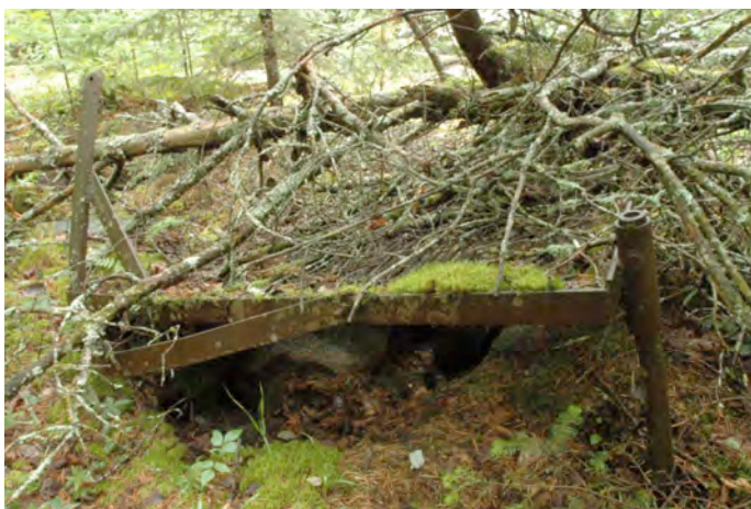
Figure 32. Logging debris, 7/13/10. Corps photo.
